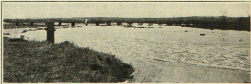
Fig. 8.—Crook river station showing river running slush ice. This flow is all seepage or return water to the river.
