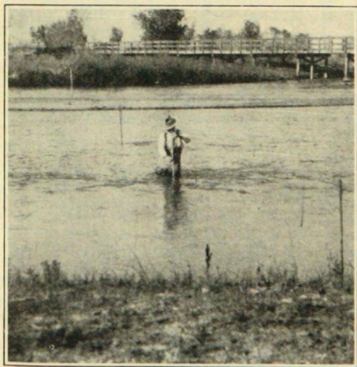
Fig. 23.—River station at Beetland showing a discharge of 300 second-feet which is all seepage or return flow to the river.
